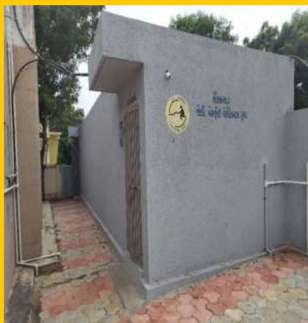
Construction of Toilet Blocks
